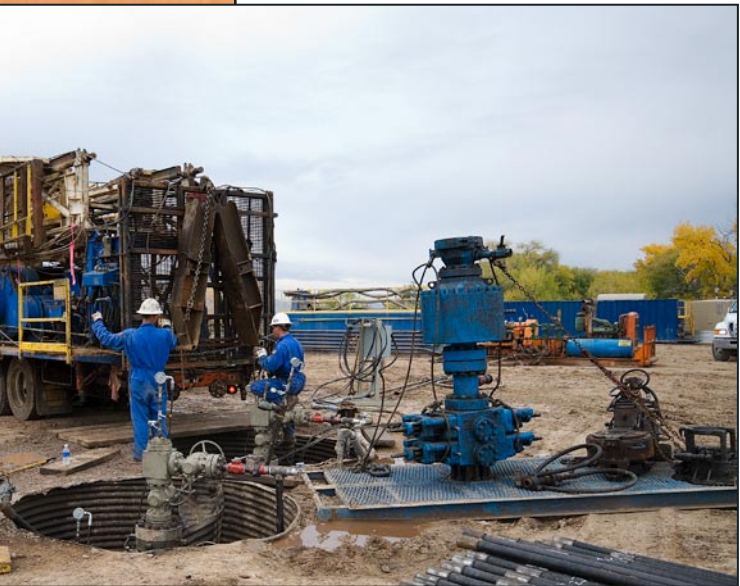
Installing the Well Head
